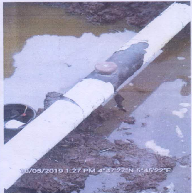
Fig D: Incident Facility during repair
