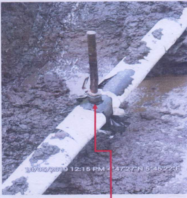
Fig C: Incident Facility shortly after excavation
